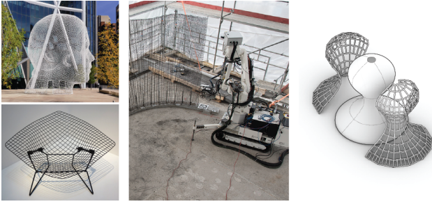
Figure 2: The 12-meter tall metal frame sculpture “Wonderland” by Spanish sculptor Jaume Plensa and the Diamond Chair design by Harry Bertoia (left). Robotically-constructed rebar for concrete applications (Mesh Mould [HLGK15], middle). Regular structures are insufficient to achieve high curvature detail, and it is unclear how to decompose complex shapes into fabricable units with globally aligned bar structures (right). Lower left image by Sandstein; license: Attribution-ShareAlike 3.0 Unported.
